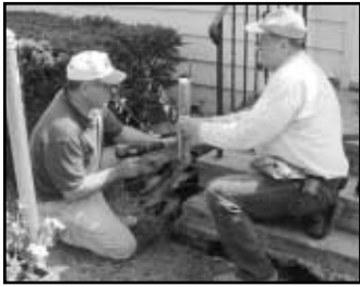
Ray Forastiero & Marvin Haun work on the entrance step renovation
